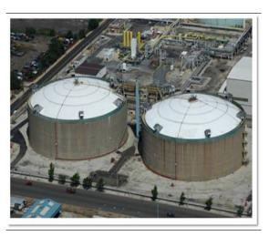
The condensation point of natural gas is -256° F. This means that natural gas, when cooled to - 256°F, changes to a liquid.
