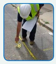
i.e. blue for water/sewer, red for electric, orange for communications to mark the location of their utility lines.
