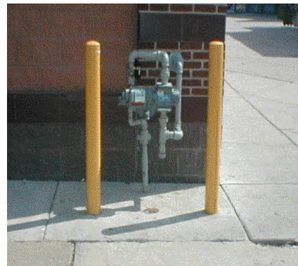
Bollards Installed to Protect
