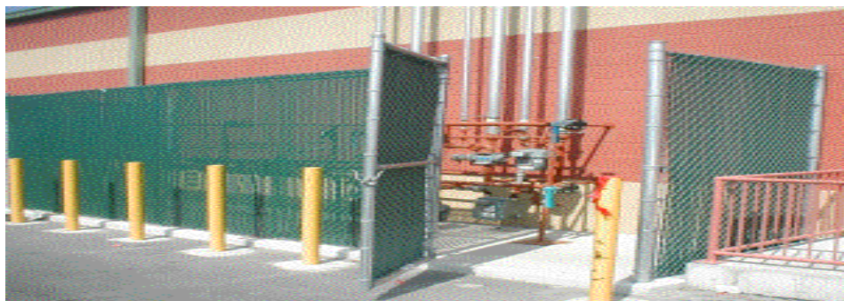
Light Commercial Multi-Metered Installation, Protected By Bollards and Fence In The rear of Shopping Center's Loading Dock.
